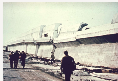
Sines breakwater failure, 1978/9
