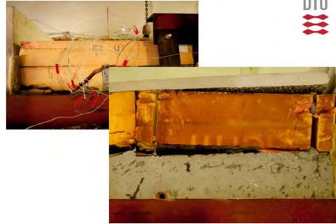
Concrete/insulation interaction showing severe debonding
