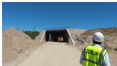
S-BRA-06, bridge supported of sheet pile walls
