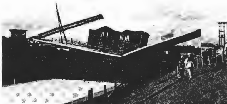
Figure 16 – Smedstua bridge after failure.
