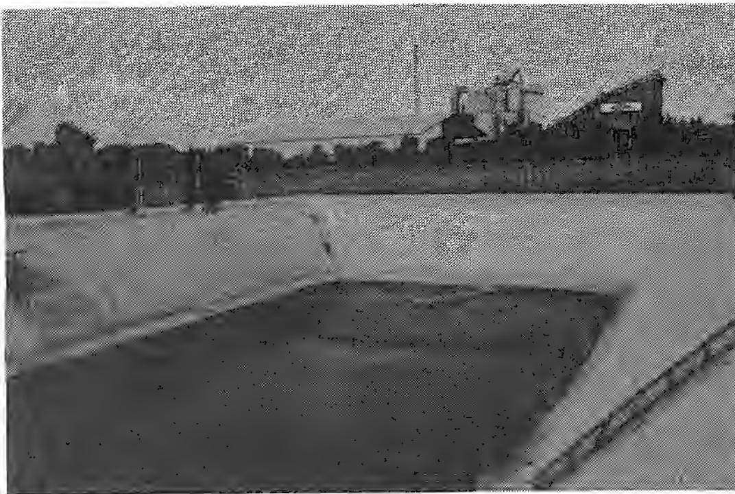
FIG. 8. Trial reservoir made with FRC
