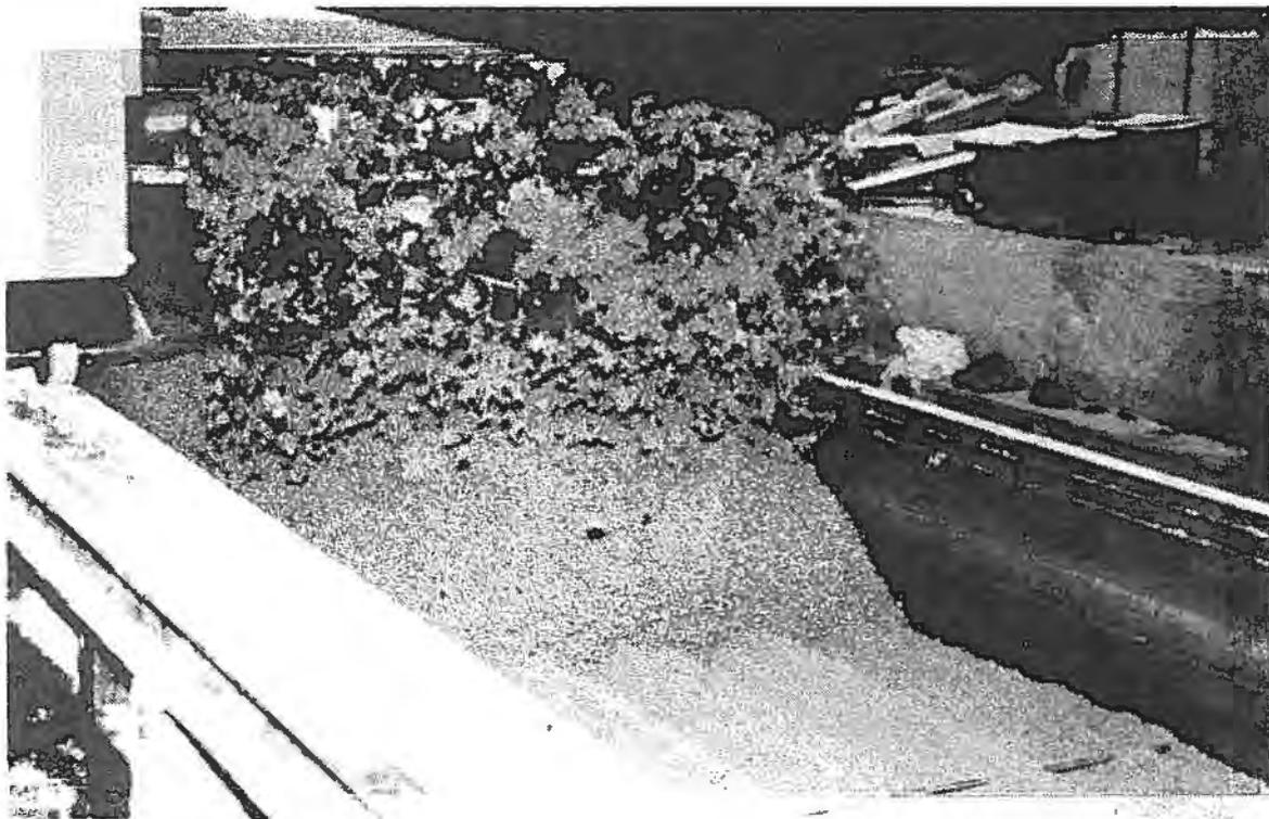
Figure 2. Placing the concrete in the form
