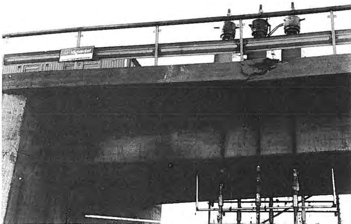
Fig. 9. Failure in the prestressed bridge. Cracking, support failure and concrete compression failure at the top of the loading section can be seen.
