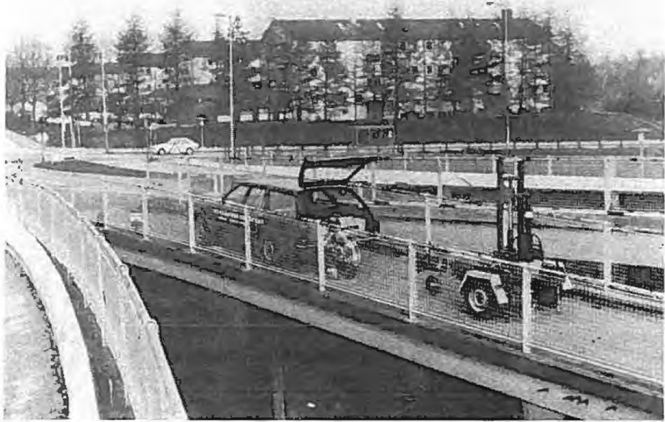
Fig. 2. Footbridge with loading arrangement.
