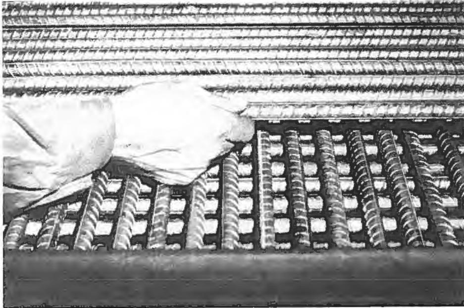
FIG. 9. Installation of reinforcement in 120 mm thick CRC plates (1100 x 1100 mm). The main reinforcement in the plane of the plate consists of 4 layers of 16 mm diameter bars at a distance of 32 mm (center to center). Shear reinforcement (not shown) in the form of bars (100 mm long, 10 mm dia.) arranged at right angles to the plane of the plates is inserted in each of the meshes in the reinforcement mats (16 x 16 mm).
