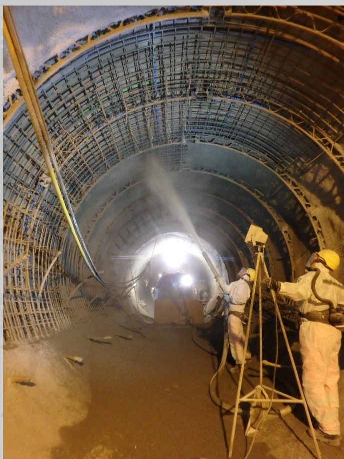
Spraying of shotcrete ring at Krauseparken
