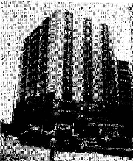
Cluster D under construction, May 1978.
